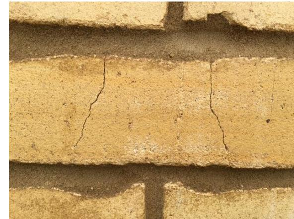
If the distance is greater than 20mm the brick should be cut out and replaced, or alternatively, filled in situ with a colour matching epoxy and finished with a colour matching sand. Well done, this should be invisible especially when viewed from the correct distance of 3M or 10ft as required by Publicly Available Specification 70. As cut and bond bricks account for over 2 out of 3 specials currently in production, there should be no concern over the use of this technology.
